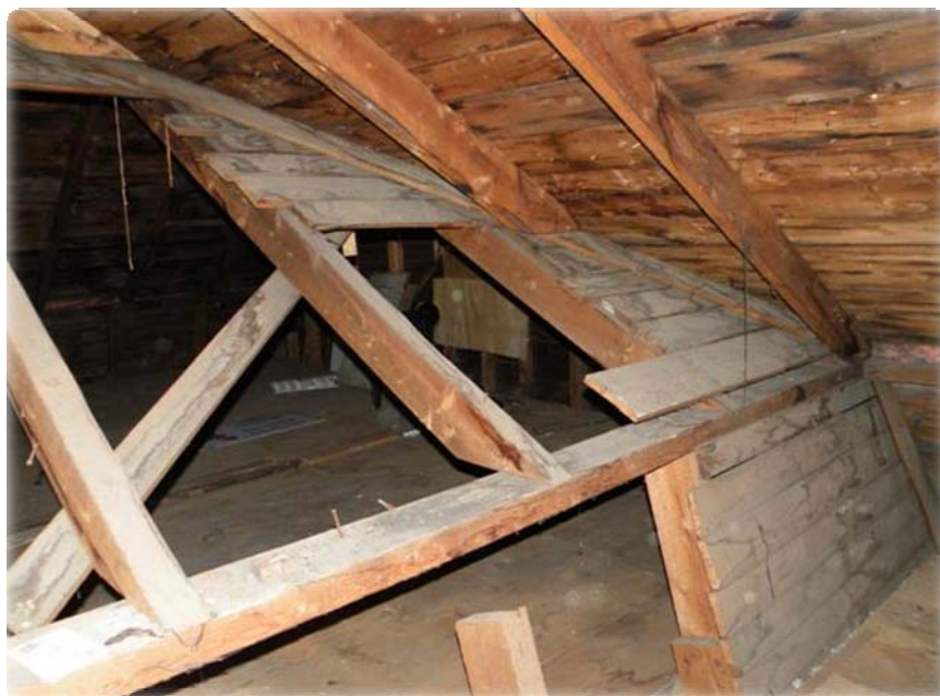
Figure 5. Interior view of the second and third roofs arching over the remnant gable of the original roof (note the original covered attic window in the centre of the image beyond the frame of the second roof).
