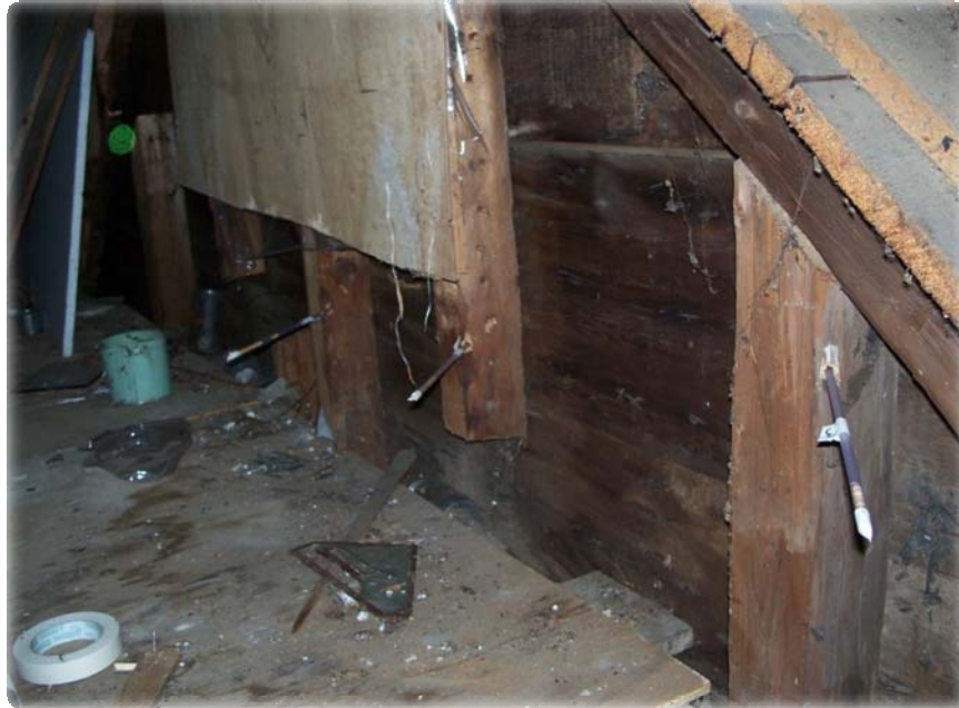
Figure 4. Samples 09ARS003, 4, and 5 taken from the south side of the attic. The image also illustrates the remnant gable end of the original roof with the sampled exterior wall beams (centre), a covered attic window (top left) and the original roof line (top right).
